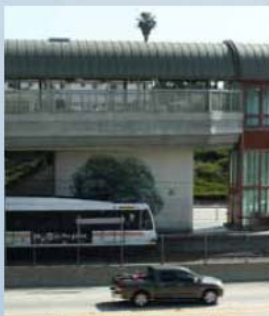
County of Los Angeles Vermont Green Line Station
