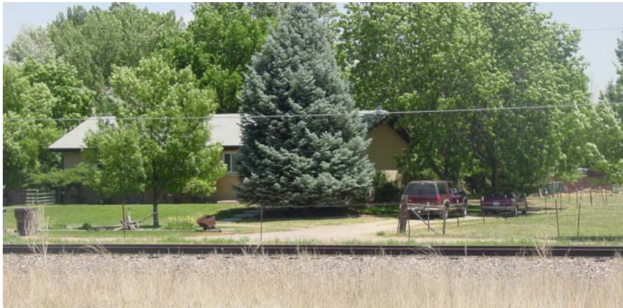
Figure ES.02-2: Residence Adjacent to the Existing BNSF Line
