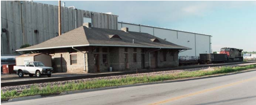
Figure ES.02-1: Longmont Train Depot Building on the Existing BNSF Line
